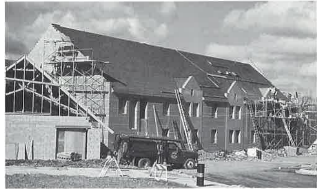
Workers complete brick and roofing on one of the residence halls.
