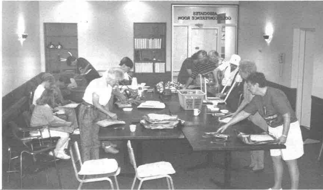
Volunteers form an assembly line to recover chairs in the renovated Associates Gold Conference Room.
