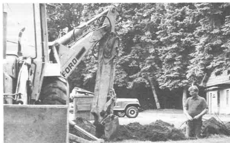
Workers install lines for the new institutional phone system.
