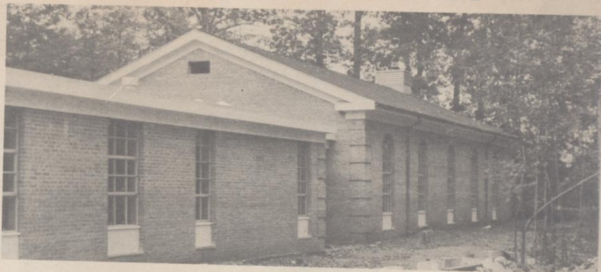
TO HERE . . . New Building 11 Mile West of Lahser
