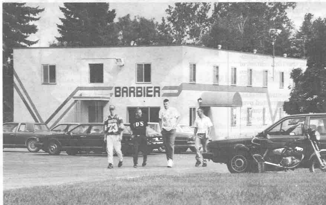
Barbier Residence Hall portrays a new image after the completion of outside renovation work.
